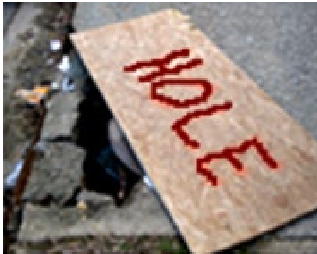
Figure 2 Plywood hole cover
